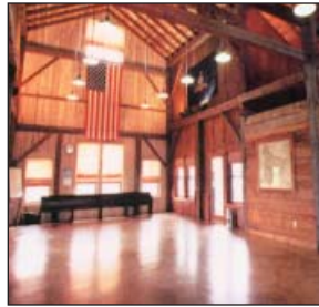
concrete floor was colored with iron oxide
