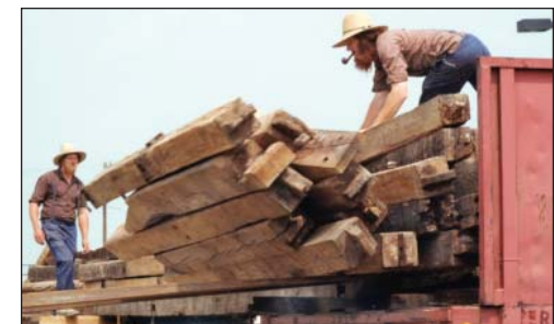
reusing original timbers
